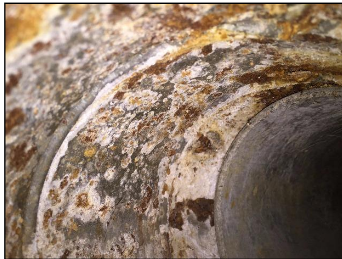
20. Rust (in-slab ducts)
