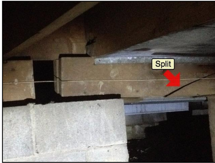
9. Rotated or twisted beams
