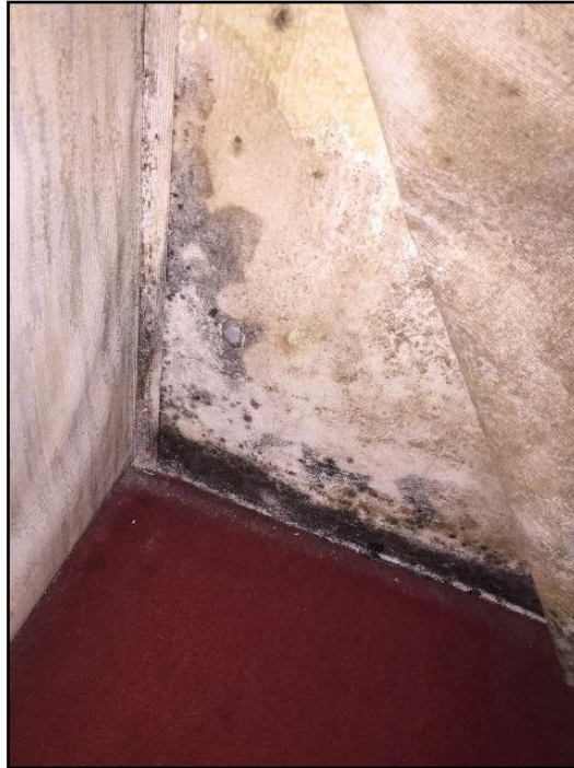
26. Water damage
