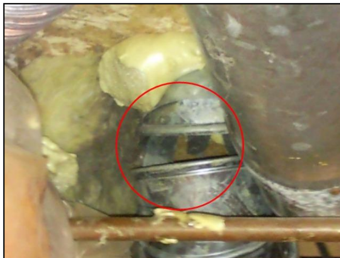
19. Disconnected ducts
