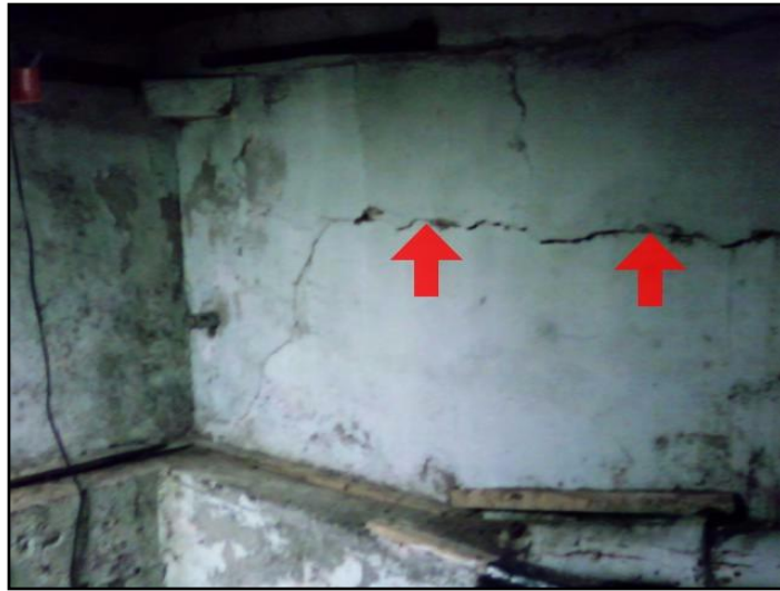
8. Cracked horizontally
